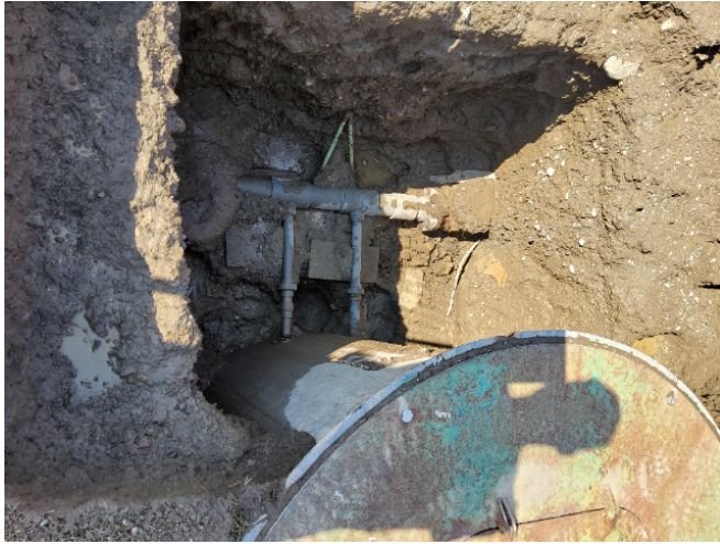
Photo 3-2: New effluent piping at Corning Preserve Pump Station
