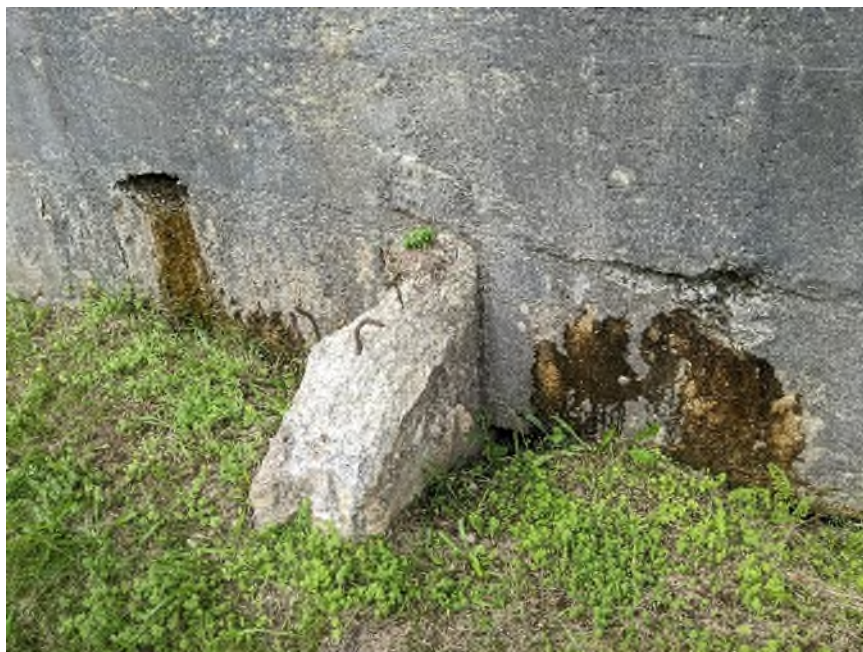
Photo 2-5. Leaking Exposed Wall in Sedimentation Basin 1
