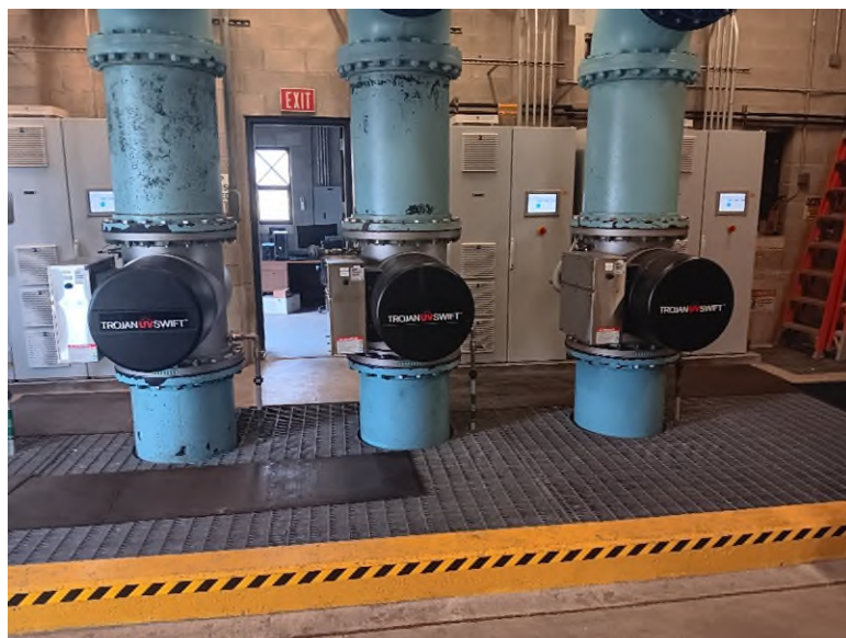
Photo 2-12. New UV Reactors in UV Building
