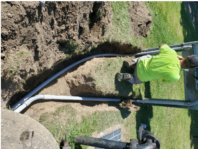
Photo 3-3: New conduit at Snow Dock
