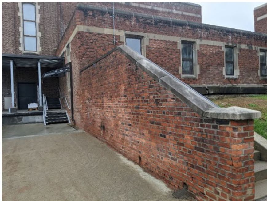
Photo 2-7. Deteriorating Brick Mortar on North Side of Building and Retaining Wall
