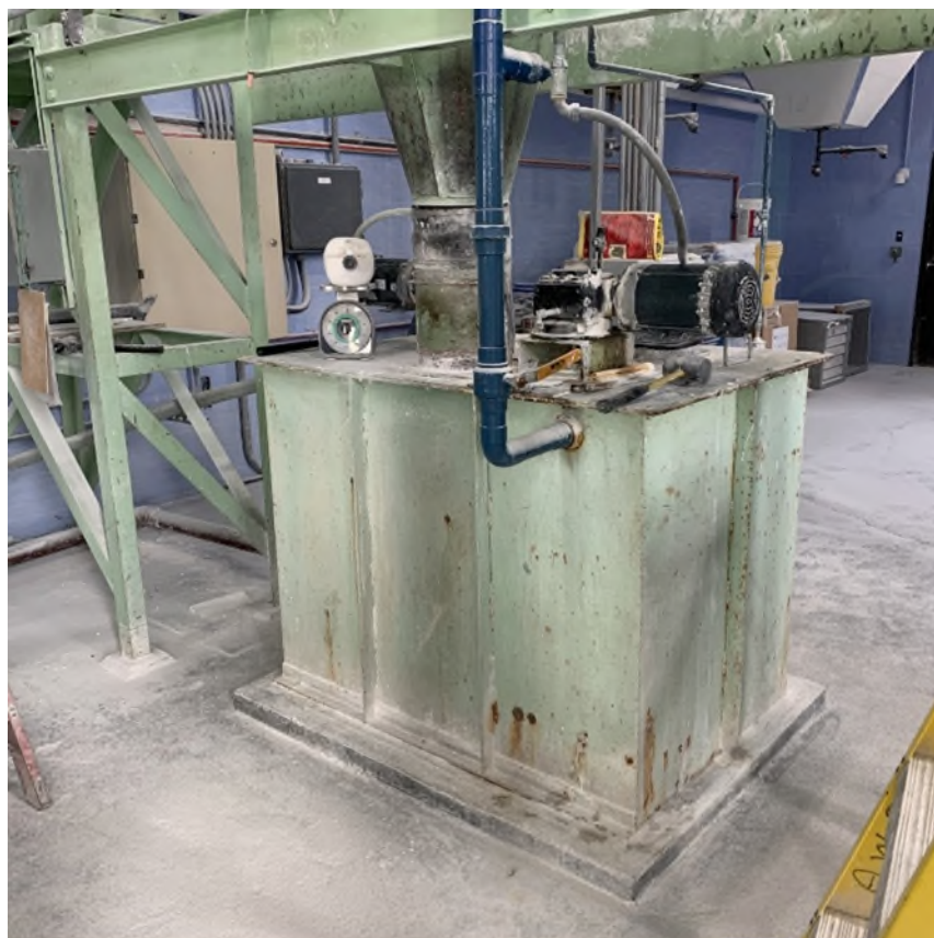
Photo 2-6. Existing Dry Lime Feed System in the Feura Bush Filtration Plant
