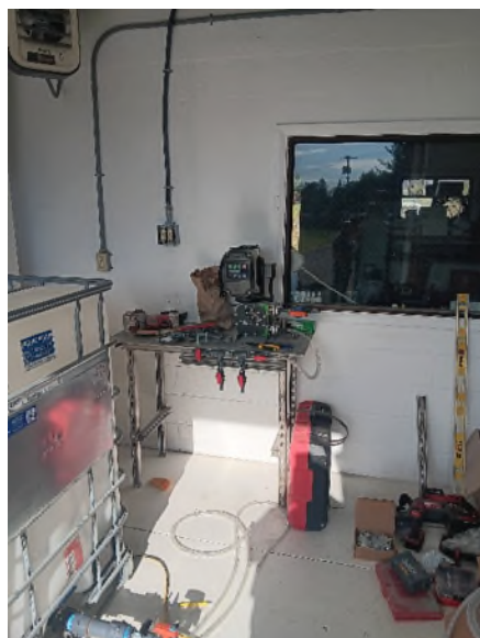
Photo 2-13. New Lime Feed System in Old Chlorination Building
