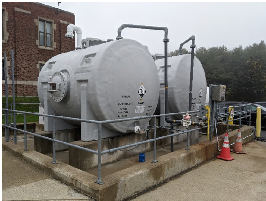
Photo 2-8. New Sodium Hypochlorite Tanks
