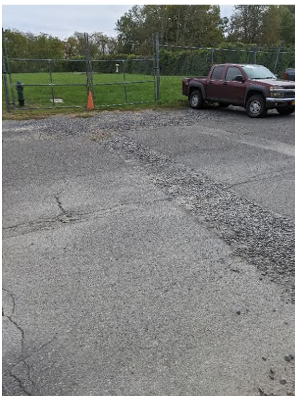
Photo 2-10. Cut/Uneven Pavement Requiring Repaving
