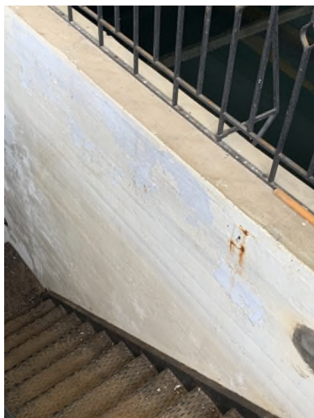
Photo 2-9. Peeling Lead Paint Leading to Filter Pipe Gallery in the Feura Bush Filtration Plant
