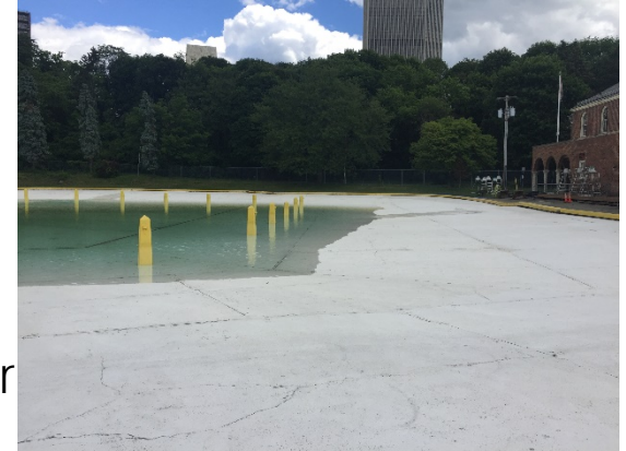
Decking Cracks
