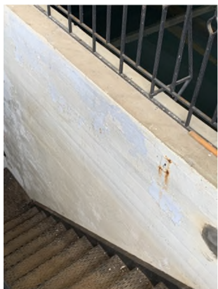
Photo 2-10. Peeling Lead Paint Leading to Filter Pipe Gallery in the Feura Bush Filtration Plant
