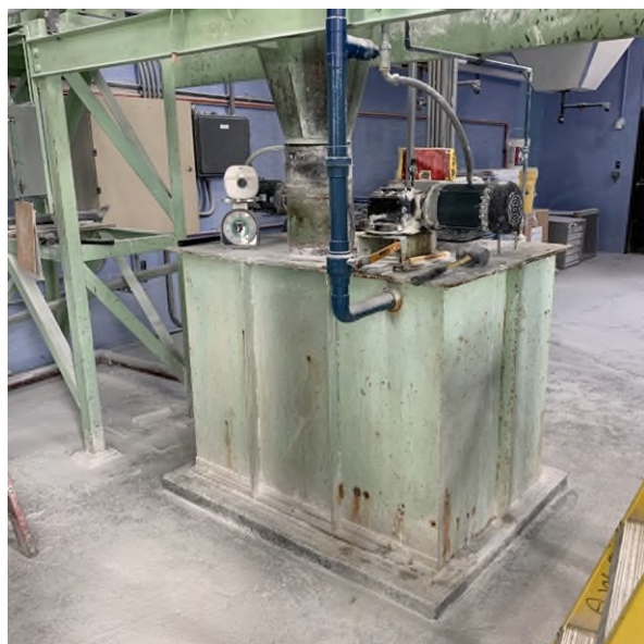
Photo 2-6. Lime Feed System in the Feura Bush Filtration Plant
