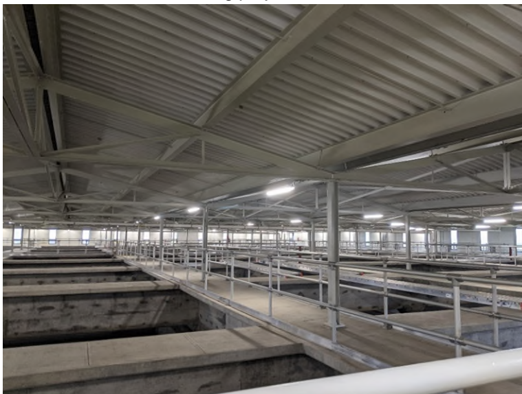
Photo 2-7. Roof Replacement Over Sedimentation Basins 4-6 Completed in the Feura Bush Filtration Plant
