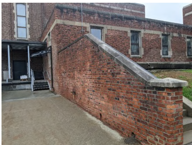
Photo 2-8. Deteriorating Brick Mortar on North Side of Building and Retaining Wall
