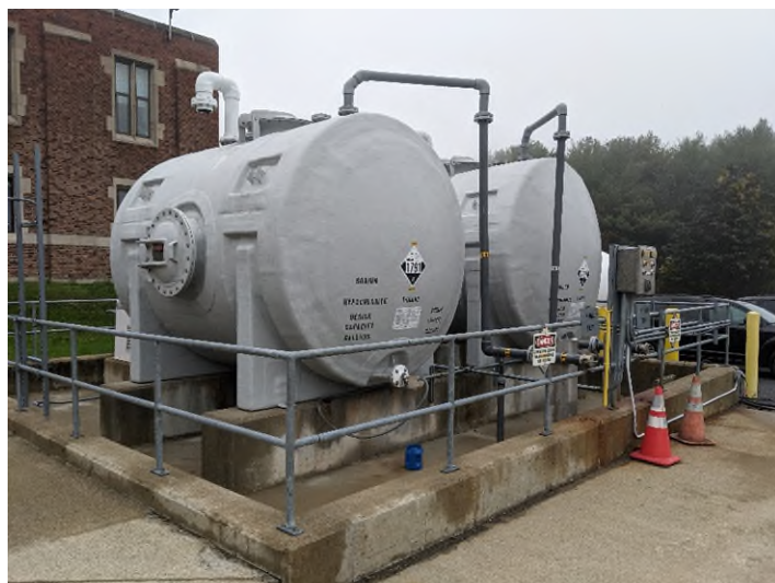
Photo 2-9. New Sodium Hypochlorite Tanks
