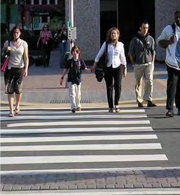
▲ Example of a high-visibility crosswalks. High-visibility crosswalks use longitudinal stripes and include continental, ladder, and zebra style crosswalks (image credit: NACTO).
