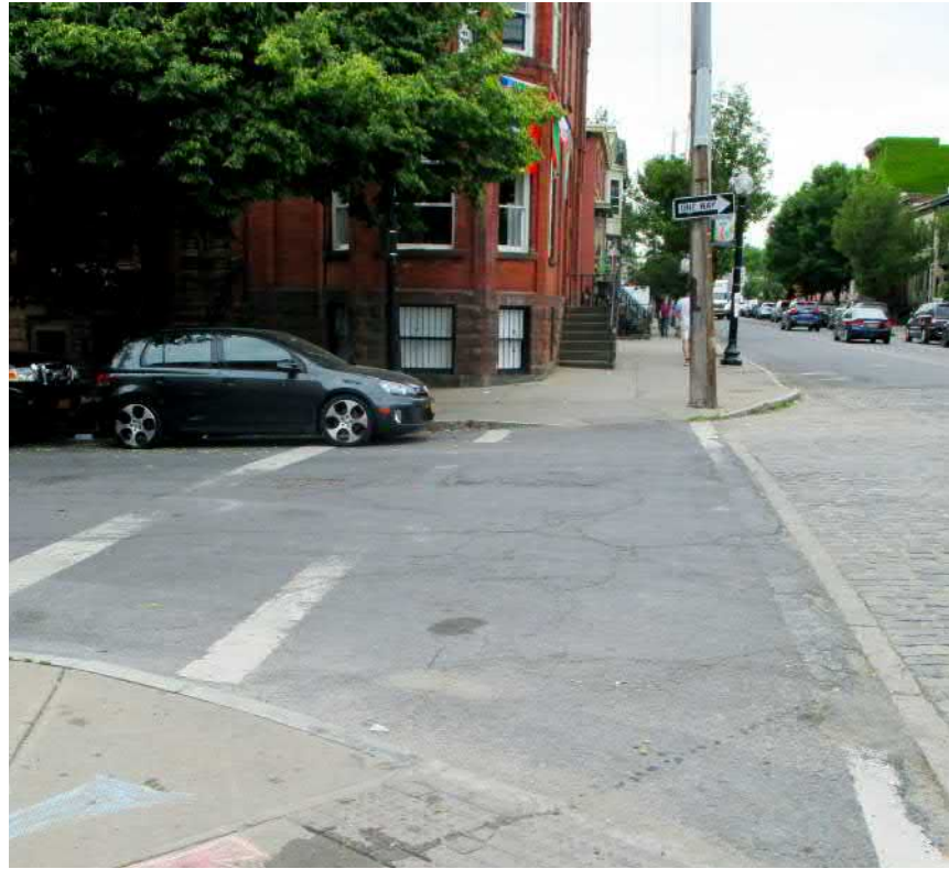
▲ A majority of the crosswalks along Lark Street are deteriorating and/or are not high-visibility (left image: Lark Street and Lancaster intersection; right image: Hudson Avenue and Lark Street intersection).
