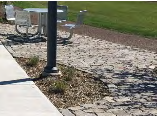
▲ Granite cobble pavers can be re-purposed and installed as pervious paving in the utility strips.
