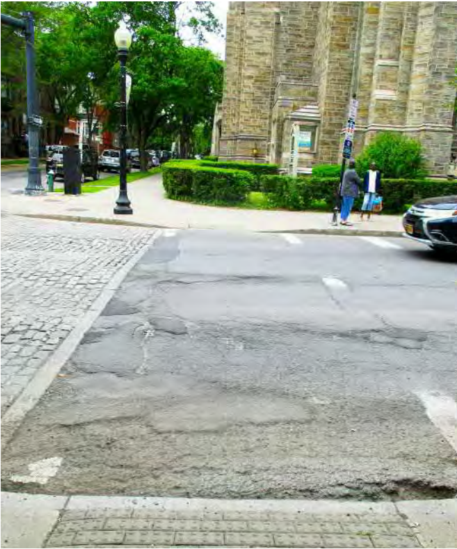
▲ A majority of the crosswalks along Lark Street are deteriorating and/or are not high-visibility (left image: Lark Street and Lancaster intersection; right image: Hudson Avenue and Lark Street intersection).
