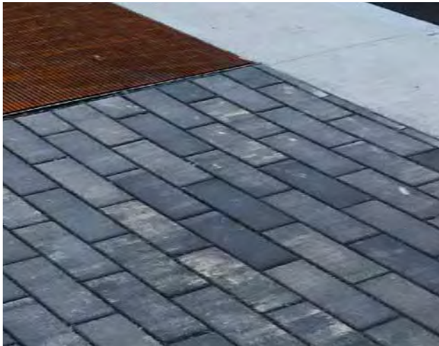
▲ Where Belgian Blocks cannot be repurposed, permeable pavers can be integrated into sidewalk spaces to increase permeability, mimic the aesthetic of the Belgian Blocks, and support accessibility.
